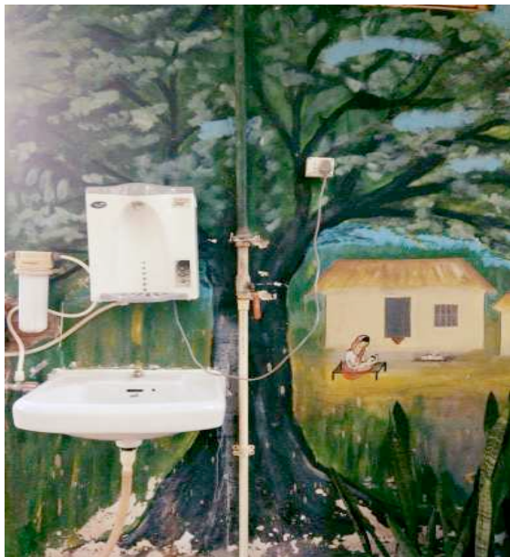
A new water filter has been installed for patients.
